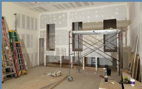
The all important frame for the screen wall is up.
