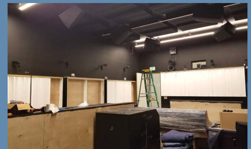
The screen wall is up and the mounts are in place. Nearly there!
